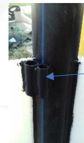
Fix with screw & clamp.
