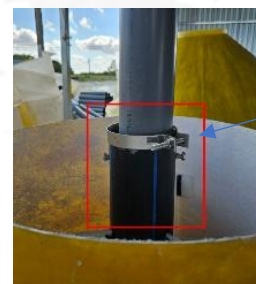
Fix with screw & clamp.
