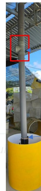
Insert upright PVC pipe into the PE pipe support
